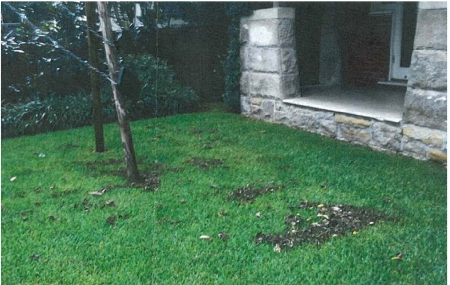
Lang Road, Centennial Park, showing settlement of leaves following flooding above height of raised front lawn.
